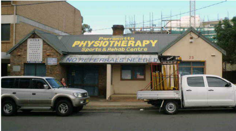
V3: Semi-detached House no.23-25 Hassall St.
