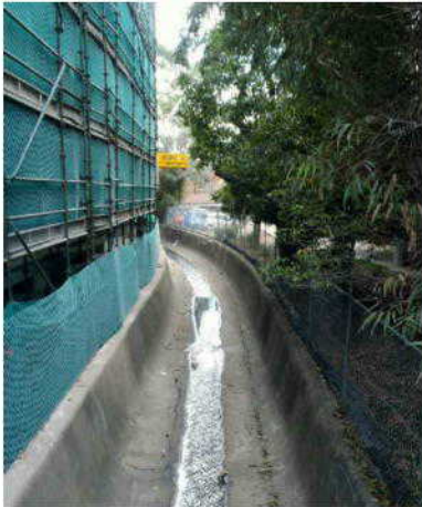
V6: Existing Stormwater Channel
